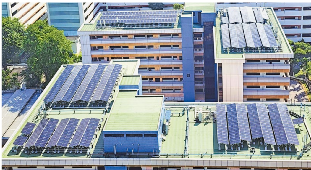
Solar panels installed at Kallang Basin 4 Cluster, as part of MIT's sustainability efforts.
