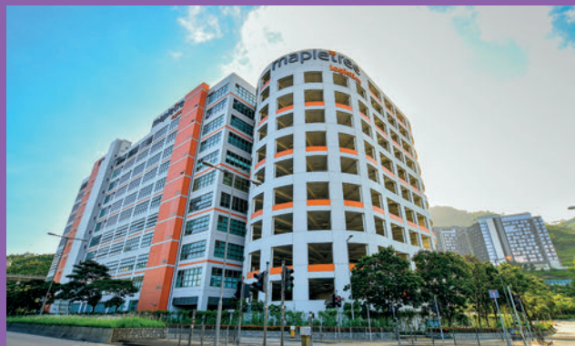
Mapletree Logistics Hub Tsing Yi
