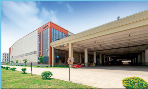
Mapletree Wuxi New District Logistics Park
