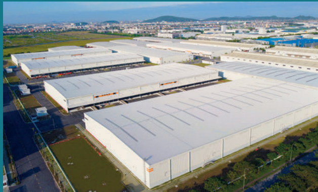
Mapletree Logistics Park Bac Ninh Phase 5
