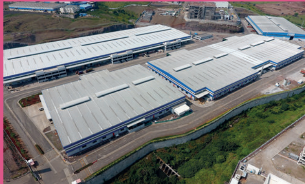
Mapletree Logistics Trust India KSH Industrial Park 1
