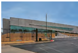
34 4121 & 4114 Perimeter Center Place, Oklahoma City
