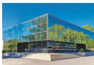
3 2601 West Broadway Road, Tempe
