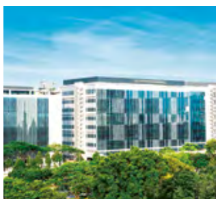
5 Mapletree Hi-Tech Park @ Kallang Way
