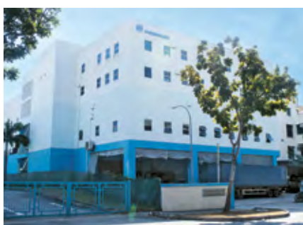
1 2A Changi North Street 2
