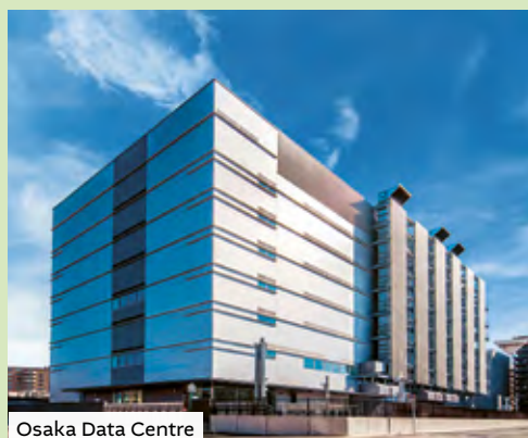
Osaka Data Centre
