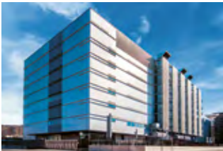
61 Osaka Data Centre
