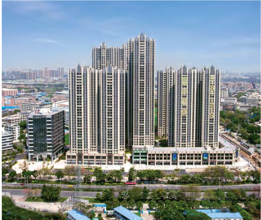
Nanhai Business City in Foshan, China, is a mixed-use development encompassing residential, retail, educational and office components.
