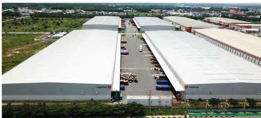
Mapletree Logistics Park Bac Ninh Phase 3, a Grade A logistics facility in Vietnam, was completed in May 2019.
