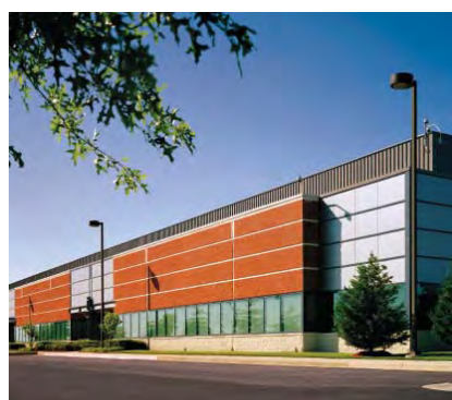
44490 Chilum Place (ACC2), Northern Virginia is one of the 13 data centres acquired in North America via a 50:50 joint venture with Mapletree Investments.
