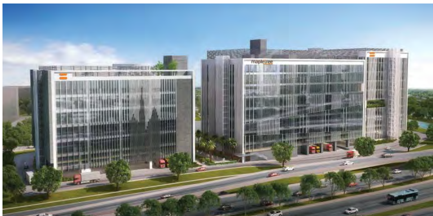
MIT embarked on its largest redevelopment of the Kolam Ayer 2 Flatted Factory Cluster in Singapore, which will increase the total gross floor area to approximately 80,420 sqm.
