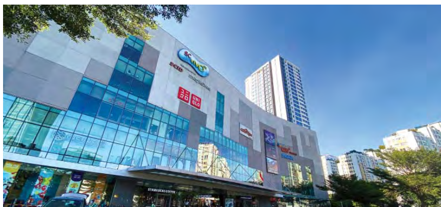
Through the amalgamation and extension of shop units and lease lines, additional NLA was created at SC VivoCity, Vietnam.
