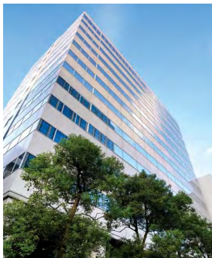
Omori Prime Building is a 13-storey office building located at Shinagawa-ku, at the fringe of the central five wards in Tokyo.
