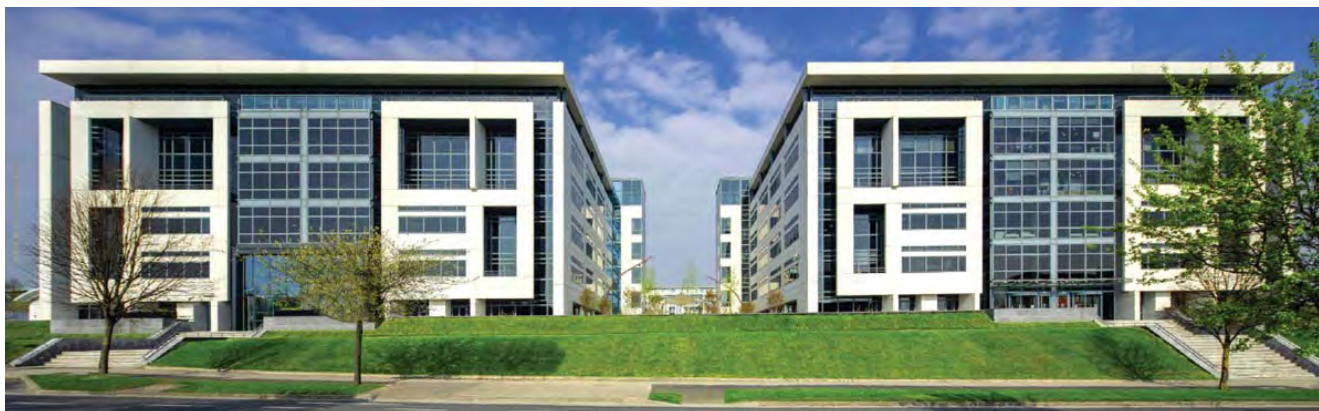
Nova Atria is located in Dublin, Ireland, and comprises two adjoining six-storey office blocks occupying 31,140 sqm in NLA.
