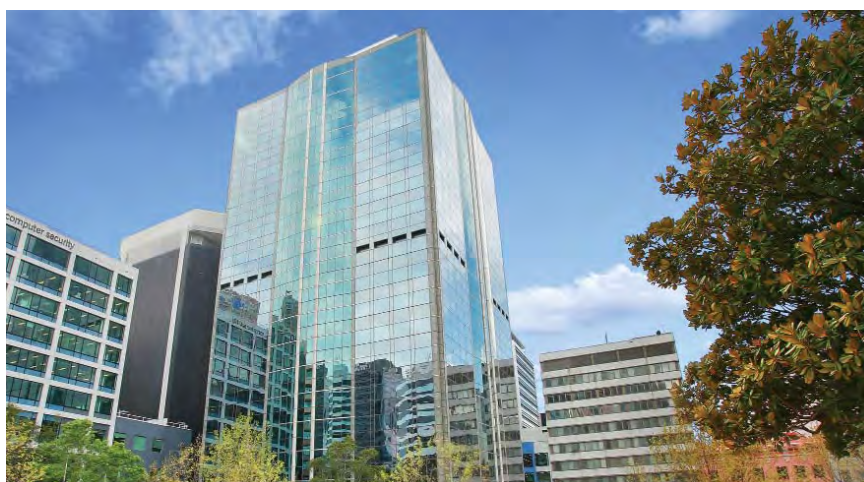
111 Pacific Highway, a 24-storey Grade A commercial building, is strategically located close to Sydney's central business district, Greenwood Plaza Shopping Centre and the North Sydney train station.
