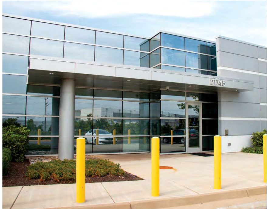
21745 Timothy Drive (ACC 9) is one of three fully fitted hyperscale data centres acquired under a 50:50 joint venture with MIT, located in North Virginia, the US.
