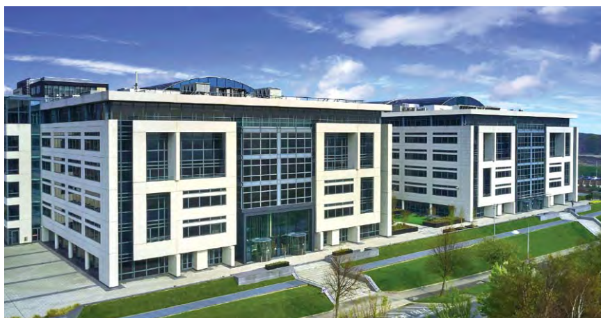
Nova Atria, located in Sandyford Business Park, Dublin, Ireland, comprises two adjoining six-storey office blocks that occupy a total NLA of 31,140 sqm.
