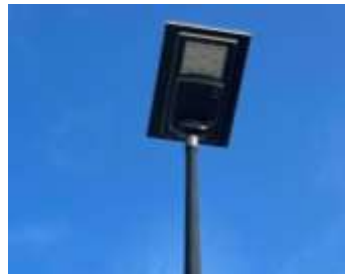
Hybrid solar LED lamp post at the Woodlands Spectrum Cluster
