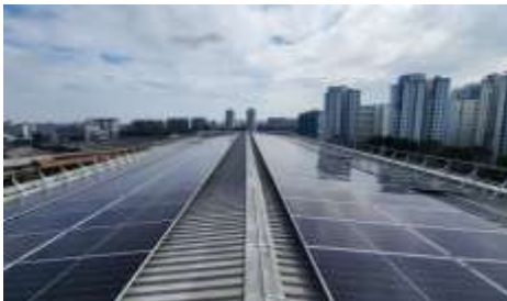
Solar panel installation at Kallang Basin 2 Cluster
