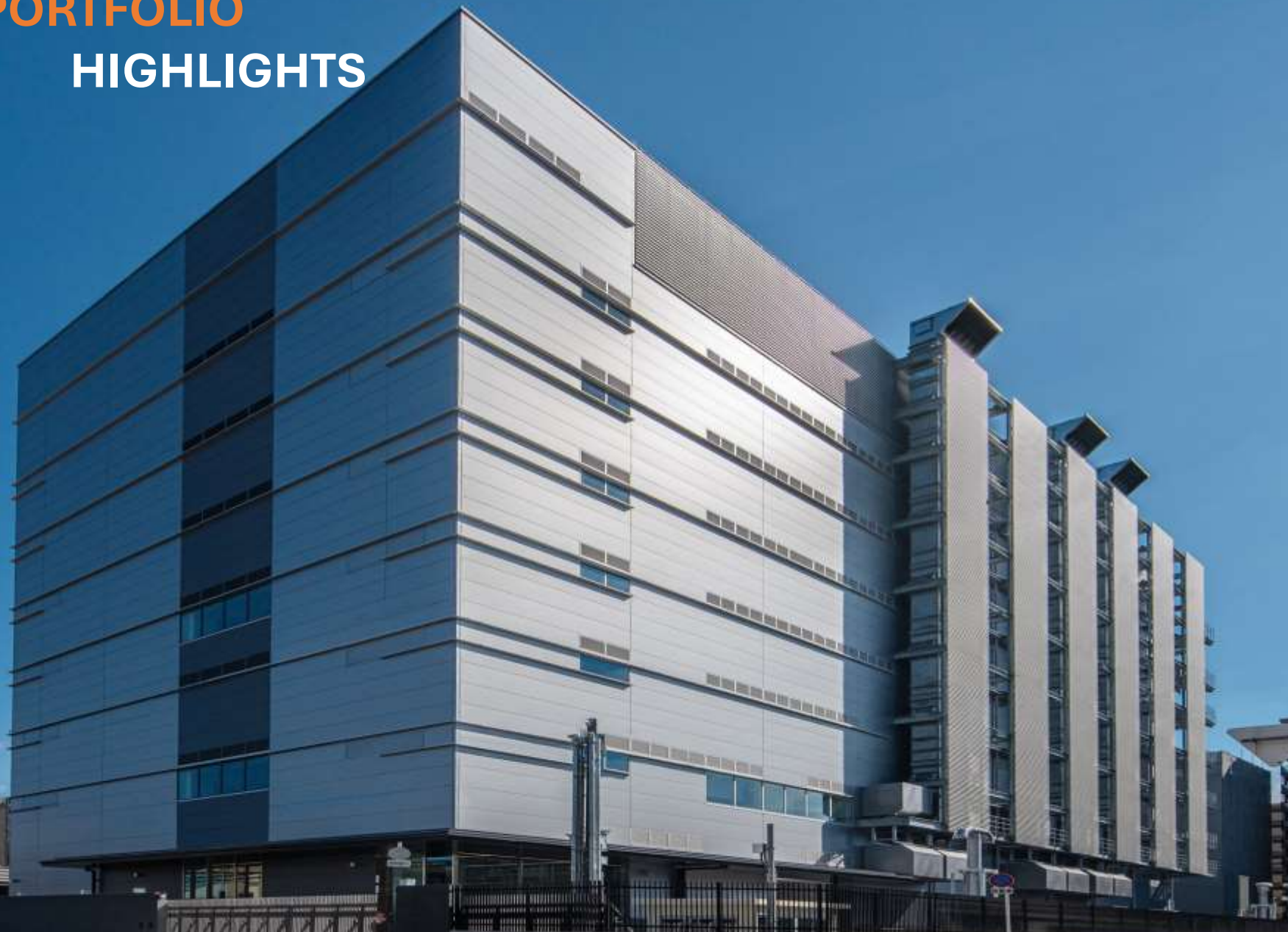
Osaka Data Centre, Japan
